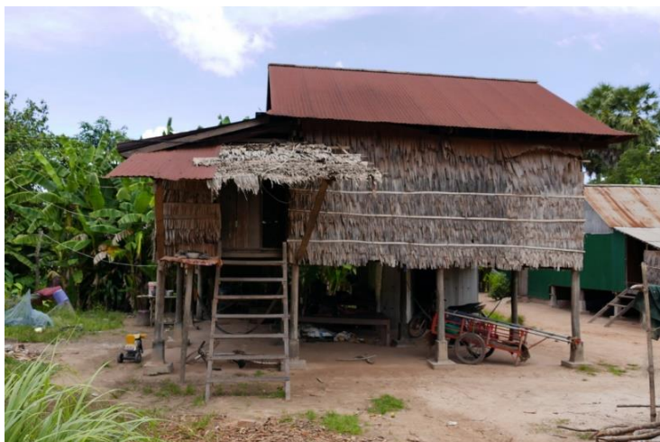
Fig. 3: Typical small house of a poorer family, built mainly from palm leaves; founded on stilts due to flooding during the rainy season.
