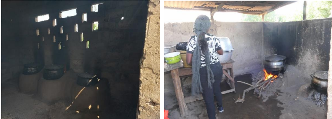
Fig. 19: The wall in this kitchen is also far too high for the smoke (heavier than air) to escape.
