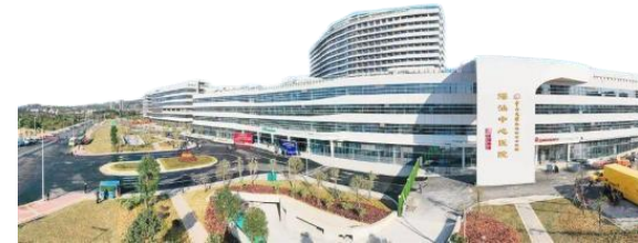
Shenshan Medical Center (Shanwei Campus Phase I)
